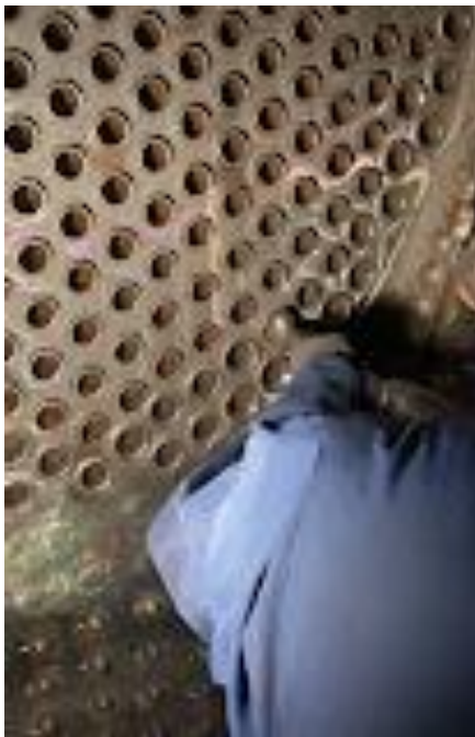
Belling over the tube ends
