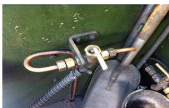
Pep (slacking pipe) valve £50
