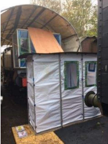
The picture on the left shows asbestos removal under way
